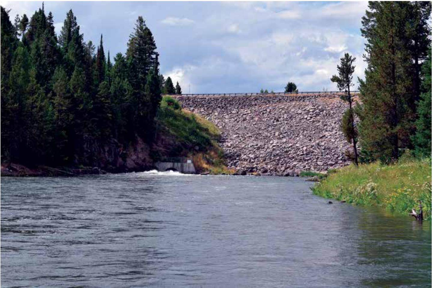
Figure 2. Island Park Dam (background) and the Henry's Fork River (foreground), showing the USBR hypolimnetic outlet on the lower-left part of the dam. Picture was taken on July 22, 2015, during peak irrigation delivery.
